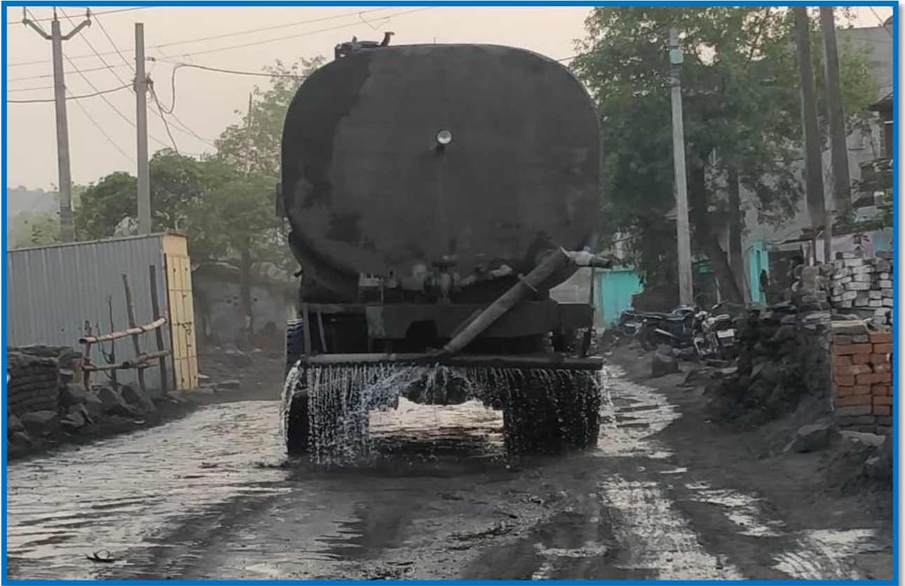
Picture 4 (I) – Water Sprinkling on Transportation Road
